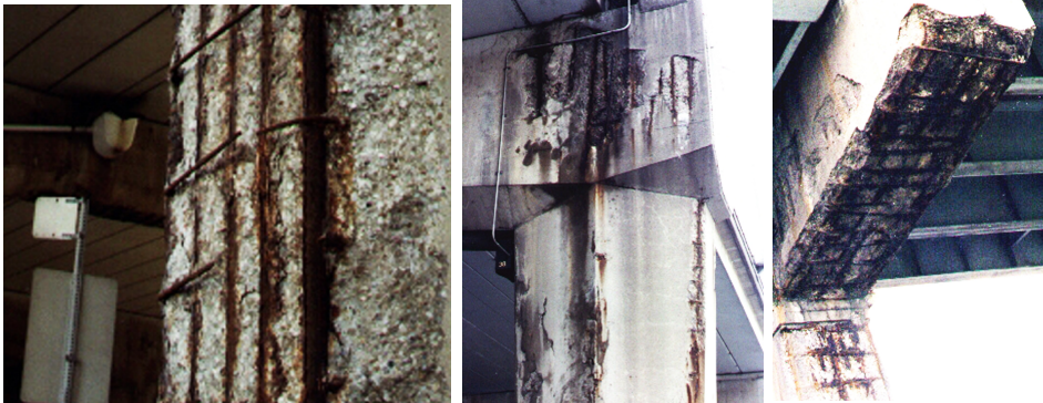
Typical corrosion of bridges and overpasses.
