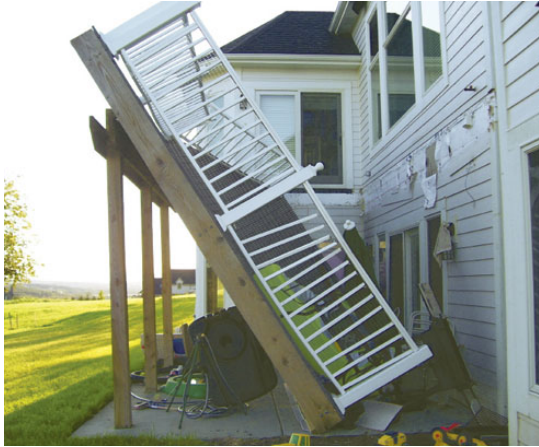
Typical deck collapse due to corroded fasteners
