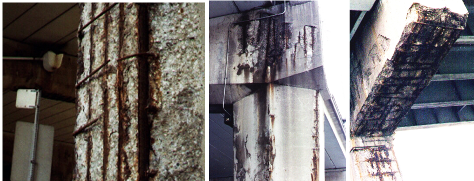
Typical corrosion of bridges and overpasses.
