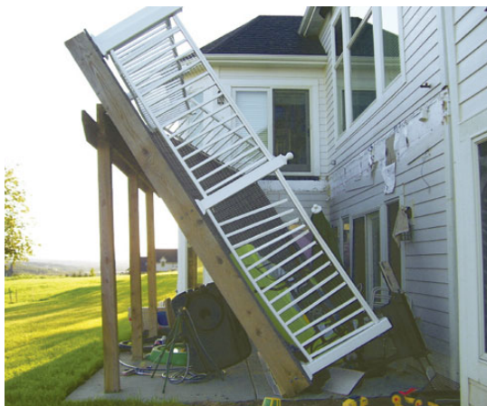
Typical deck collapse due to corroded fasteners
